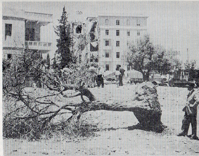
Zionist bombing of the Mandatory Government H.Q. in the King David Hotel in Jerusalem, on the 22nd of July, 1946.
